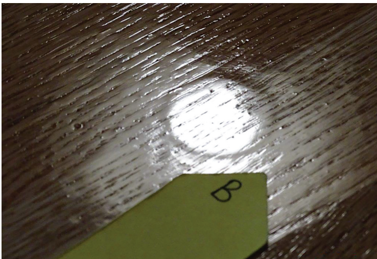
This drip was one of many finish flaws on this insurance job.
